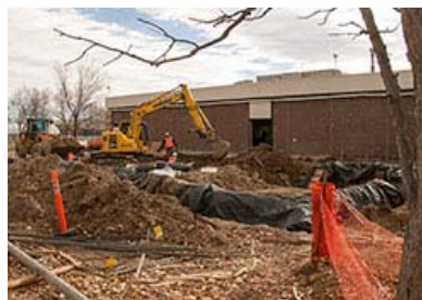
Mount Antero under construction.
